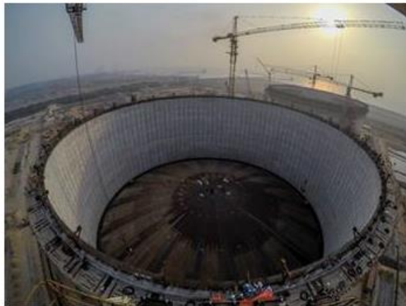
Initial aerial view of tank roof before air raising.
