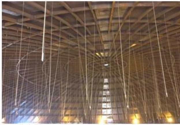
An inside view of LNG Tank Roof before being raised.
